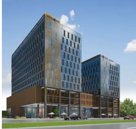
left and opposite page: stage 1 of the "Alchemia" office-service park in Gdańsk www.alchemia.gda.pl
